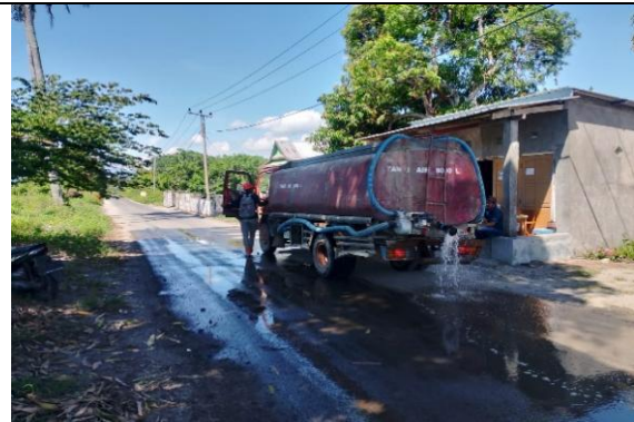
Road Watering to Reduce Dust
